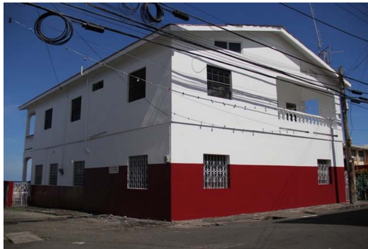
Building that will house the Health Services in Gouyave
